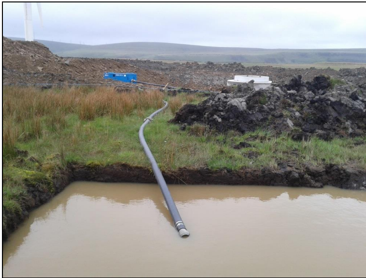
Plate 6: Typical 'Siltbuster' and settlement lagoon
