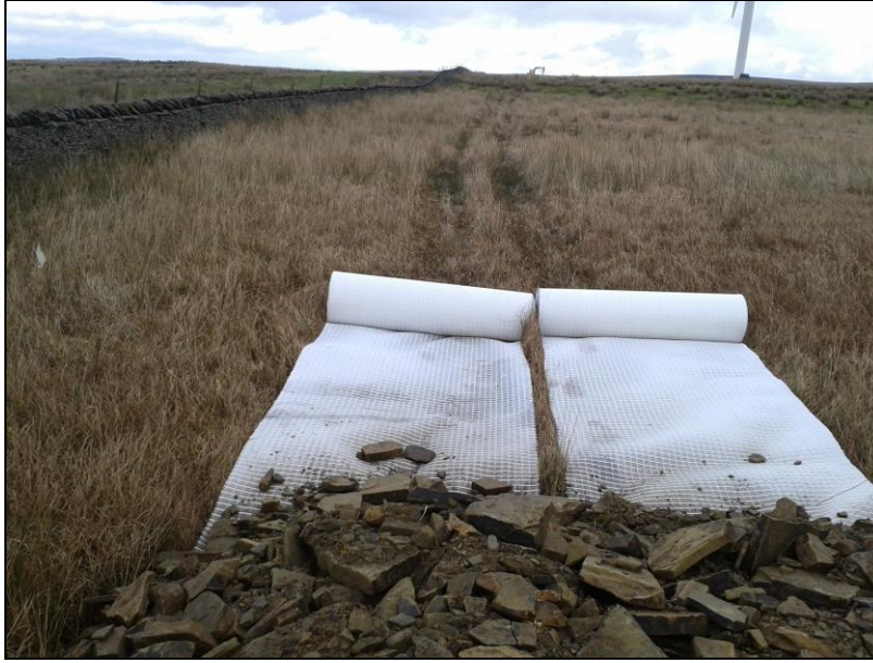
Plate 13: semi-permeable geotextile layer
